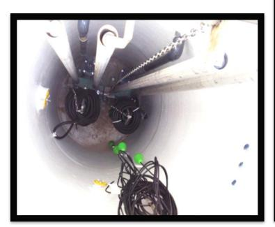
Photo 2: Shows the plug and check valves with support brackets each side.
